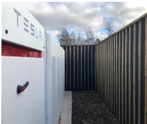
Enclosure - Security and Acoustic Fencing
